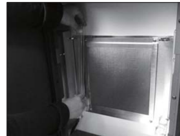
6-8 Hold the UV LAMP, pull it up remove it from UV LAMP holder.
